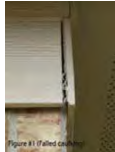
Figure 1 (Failed caulking)
