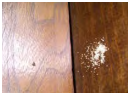
Drywood termite fecal pellets.
