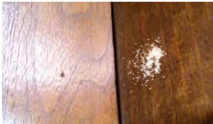
Drywood termite fecal pellets.
