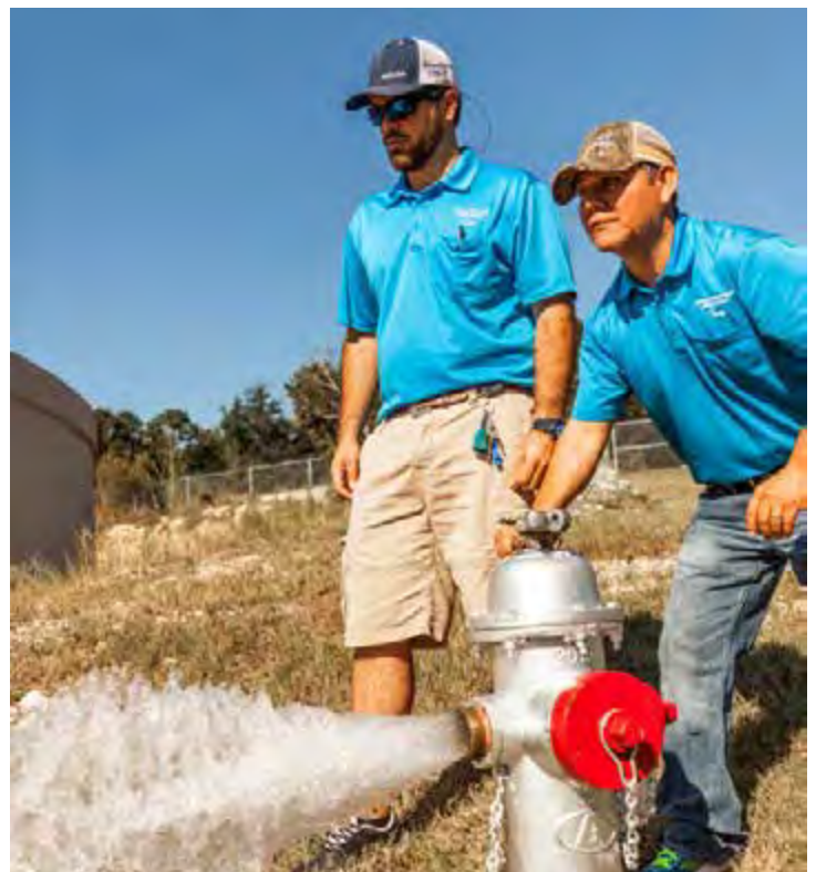
Kyle Wilds II and Tony Resendiz from Lakeway MUD perform routine hydrant flushing, an important, controlled procedure to help maintain water quality.
