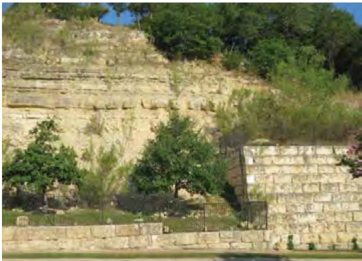
Photo of a good exposure of the Upper Member of the Glen Rose Limestone in Lakeway, Texas. This photo was taken on Highland Boulevard. It shows a very thick road cut of this formation. Note the large dimension stones in the foreground (retaining wall attributed to Cordoba Cream).
