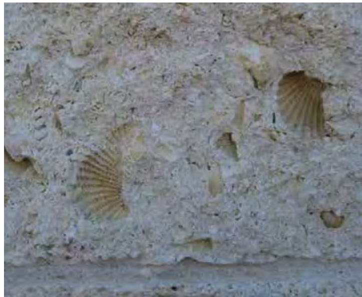
Close-up photo of “Cordoba Shell” dimension stone showing the many voids left by the impressions of marine invertebrates. This photo was taken at the Target store nearest to Lakeway, 3702 Ranch Road 620 S., Bee Cave, Texas.
