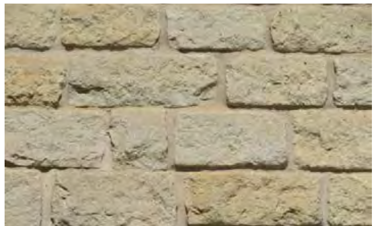
Photo of typical “Cordoba Cream” dimension stones used as a facade to a home in Lakeway, Texas, as is very common in our community.
