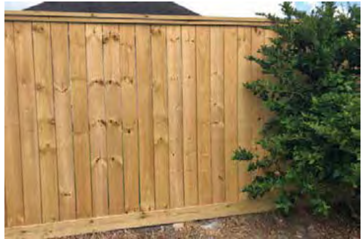
Fence with six-inch rot board at the base, six-foot picket, and two-inch header.
